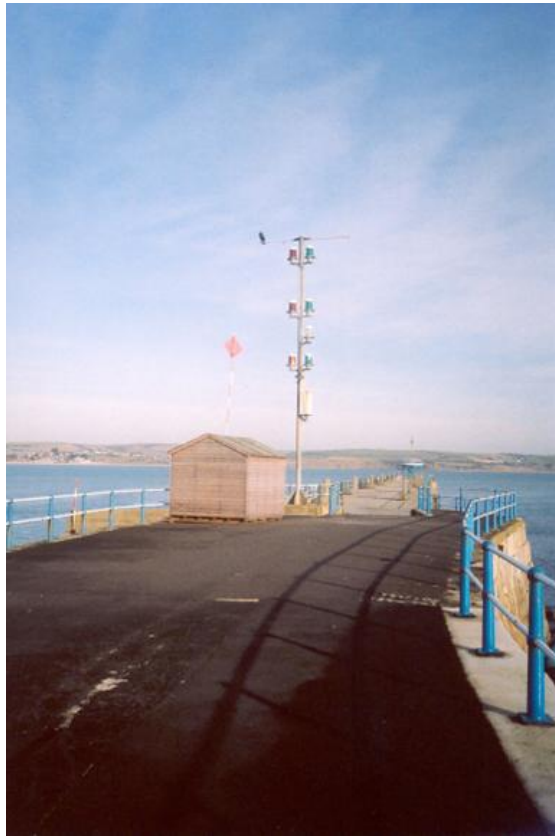
Figure 16: Movement control signal tower on South Pier end
