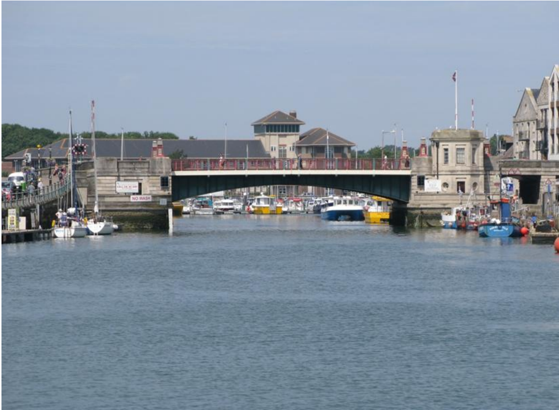
Figure 14: Town Bridge closed
